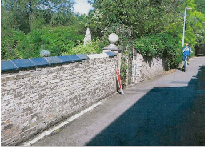
Wall prior to demolition
